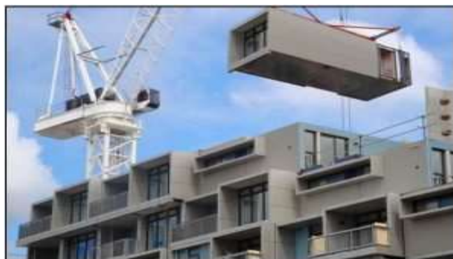
Fig.14.4 3D volumetric construction
