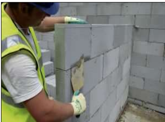
Fig.14.10 thin joint masonry
