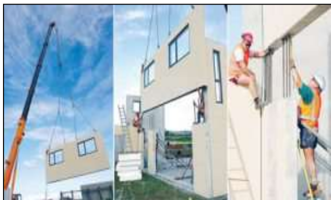
Fig.14.5 precast flat panel modules
