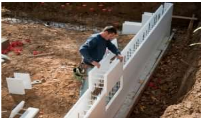
Fig.14.11 insulating concrete formwork (ICF) technique
