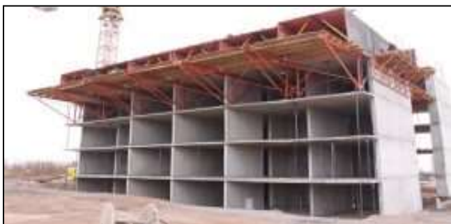
Fig.14.6 tunnel formwork system
