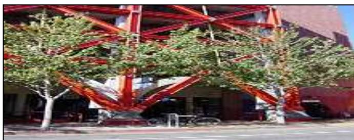
Fig.14.3 massive exterior structure
