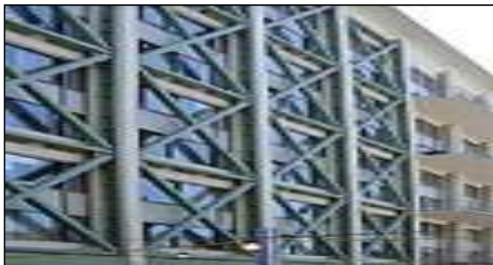
Fig.14.2 infill shear trusses
